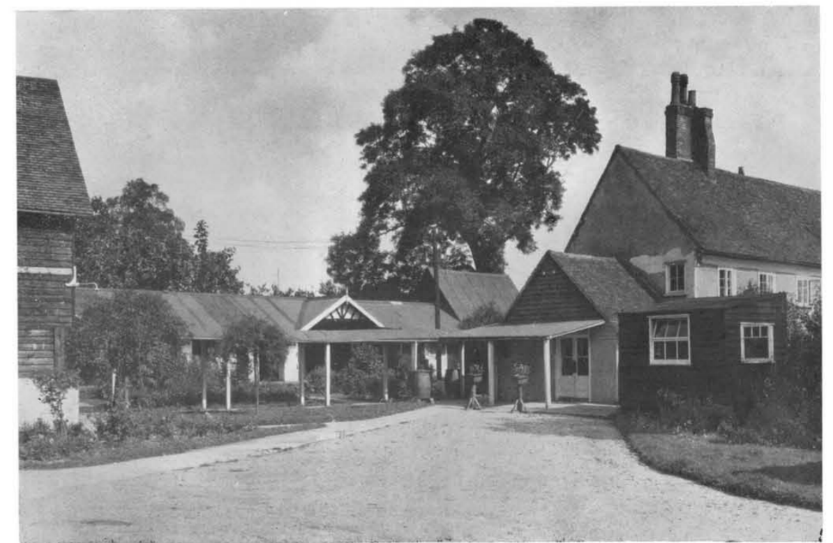
Malting's Farm Sanatorium.—The Courtyard.
