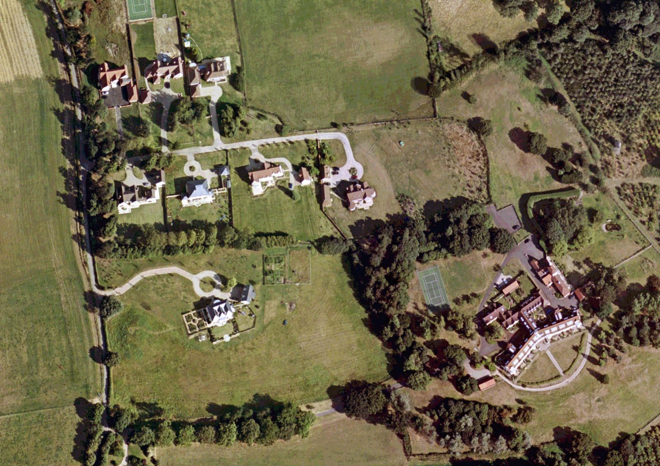
Aerial view of Jane Walker Hospital, Wissanton c.2001
